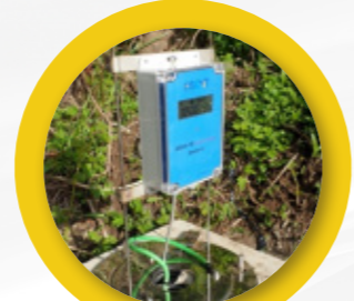
Jeju Bollard installation
