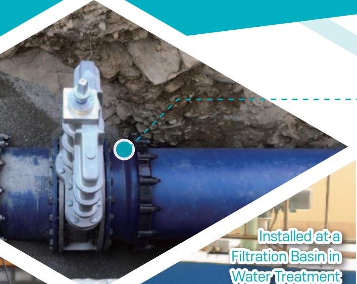
Nongong 1 Booster Station Drain Pipe Rehabilitation 600A
